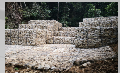
NECC Upgrading Project, Kuala Gandah, Pahang
